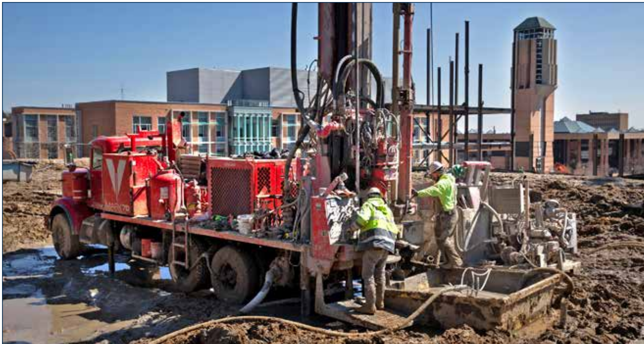
Figure 05. Geothermal drilling on Hayward Street
